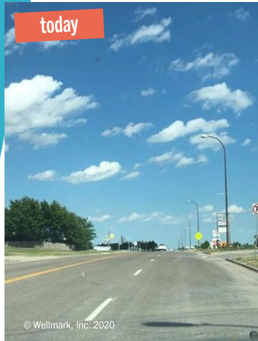
Safety on Highway 18 could be improved by implementing a road diet.
