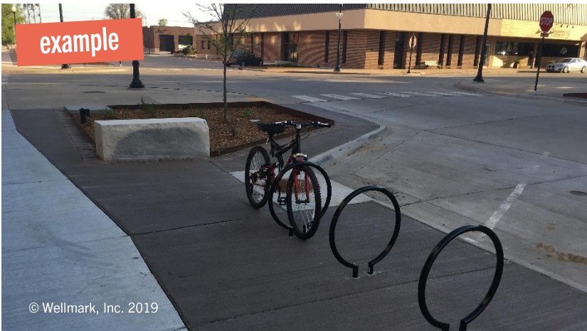
Downtown intersections in Martin could be enhanced by constructing bumpouts like this example from Yankton, South Dakota.
