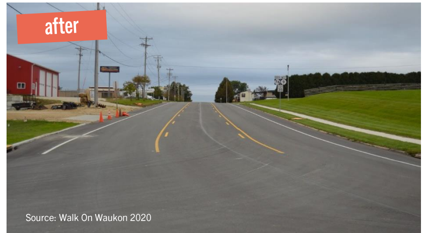
Example of a road diet implemented on a state highway in Waukon, Iowa.
